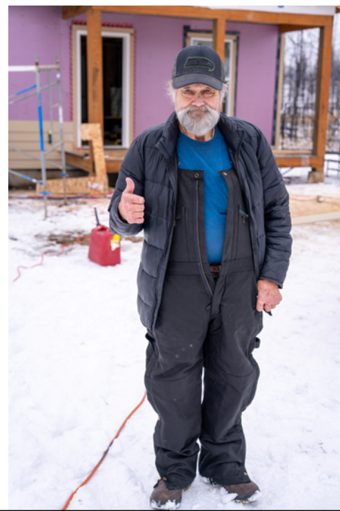
Elk resident Steve Van Buskirk shows appreciation for the new house MDS volunteers are building for him.
